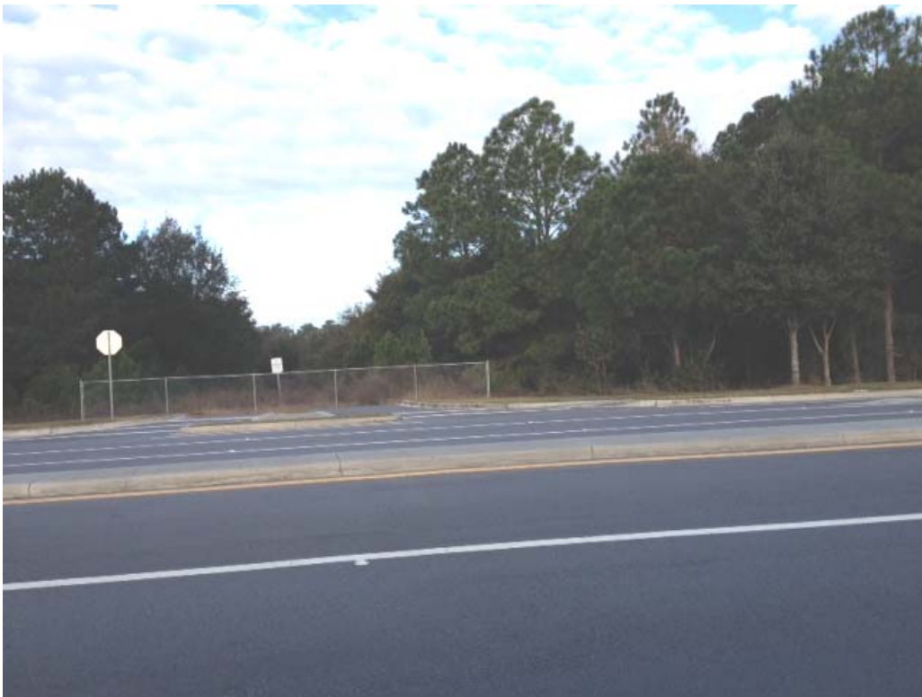
View of existing curb cut on Kendall Drive.
