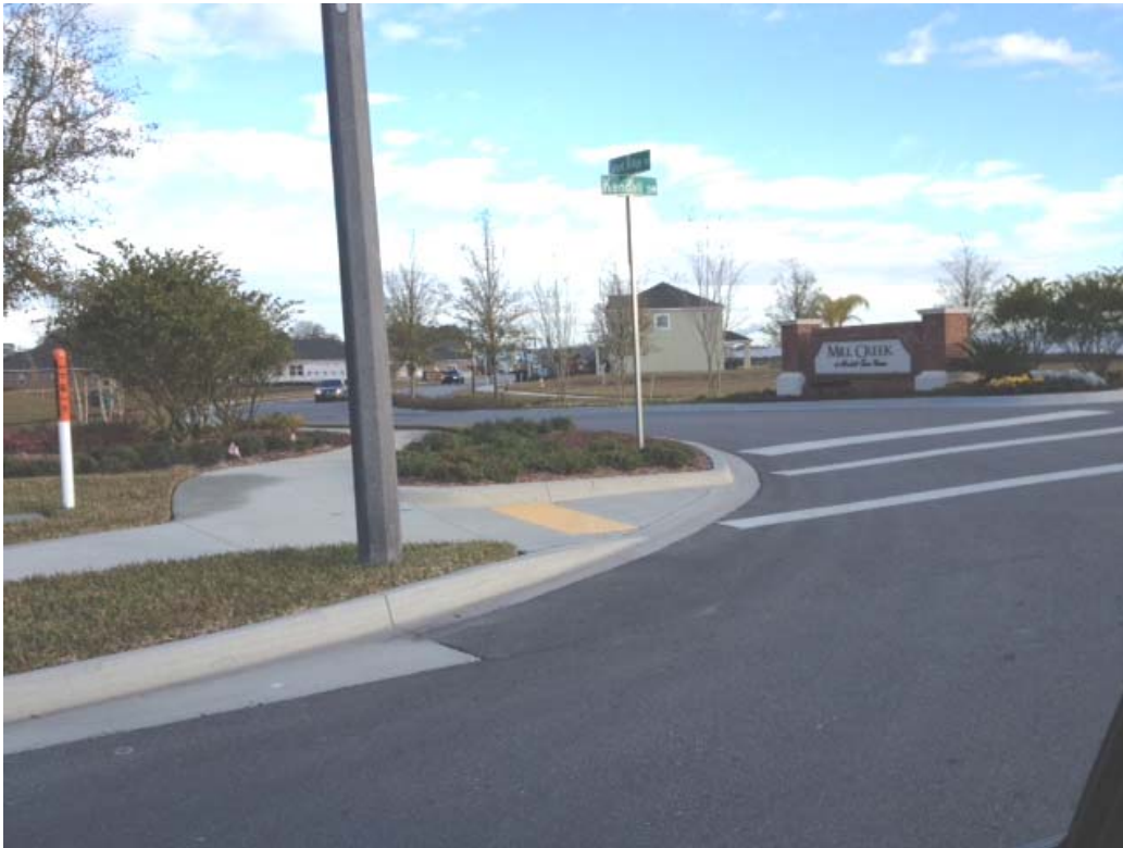
Entrance to Mill Creek subdivision.
